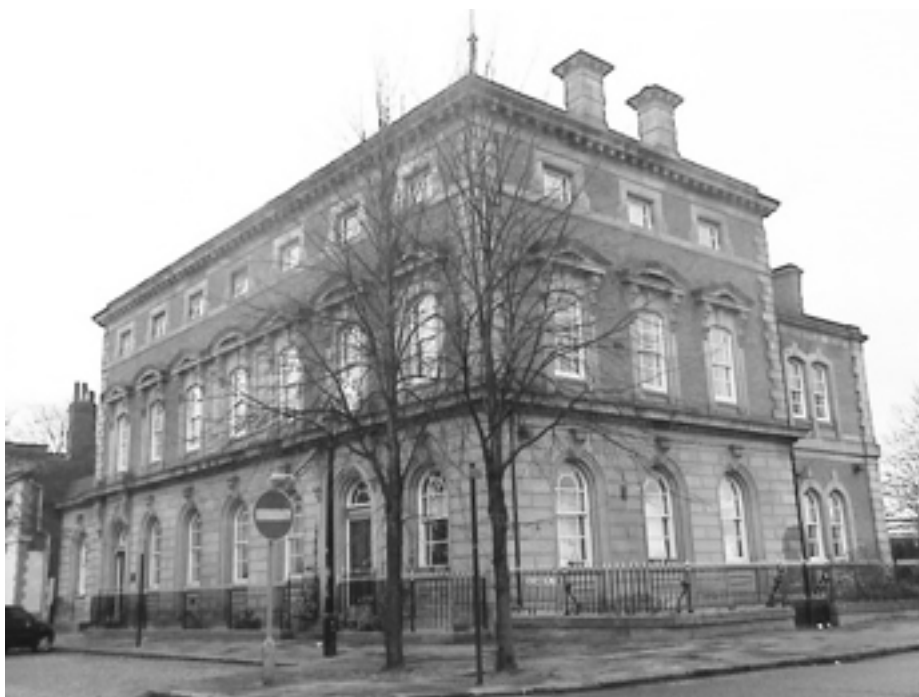
County Courts, Encombe Place, Salford (c.1865).
