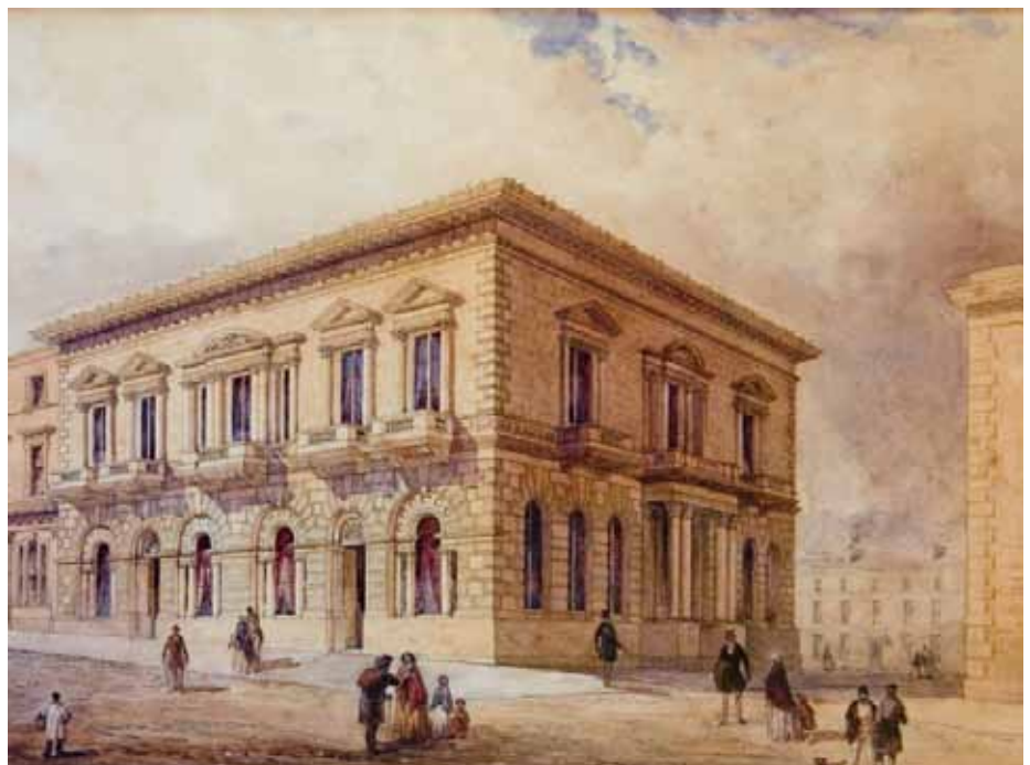
Burnley Mechanics Institute (1854-55) architect James Green
