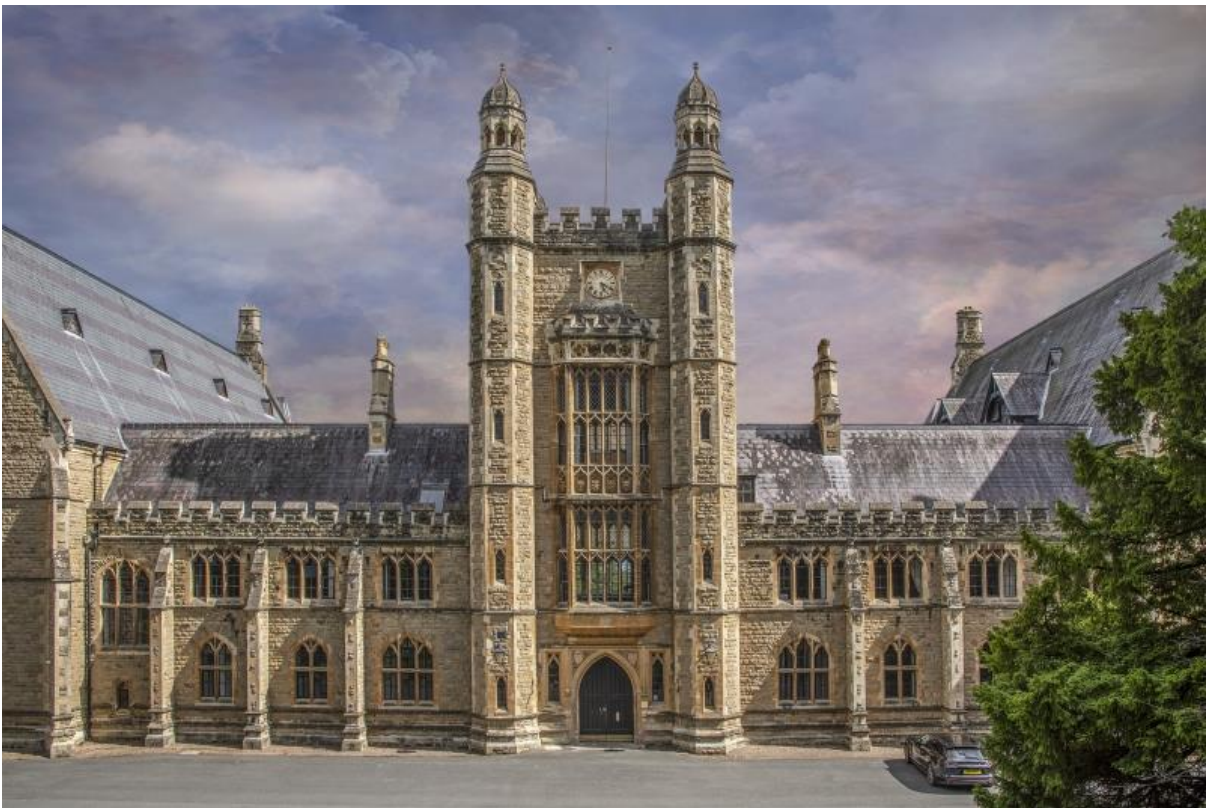
College main building (from College Road)
