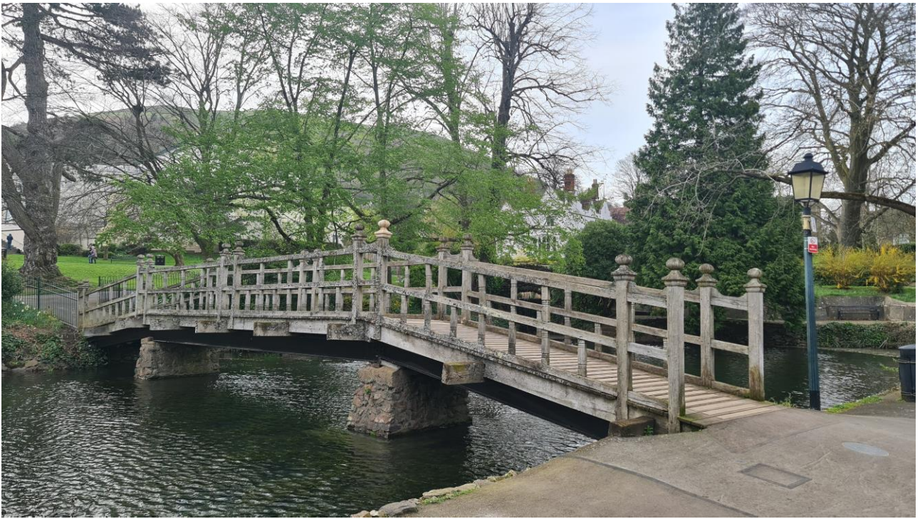
PRIORY PARK BRIDGE
